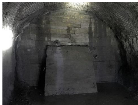
(a) Concrete rigid retaining wall
