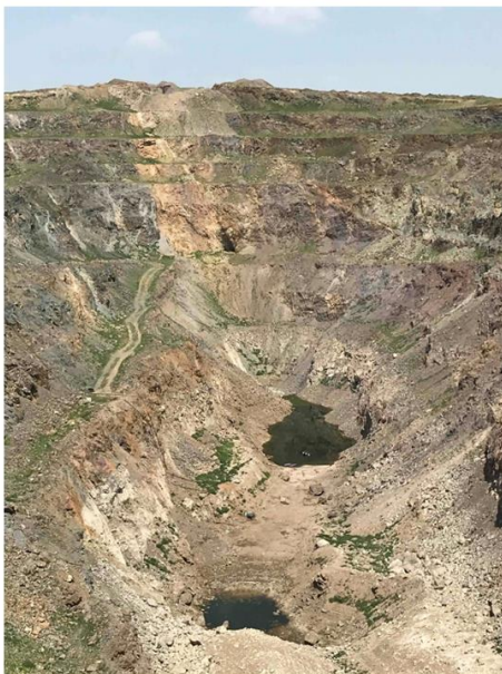
Figure 3. An overview of the open pit (note the fault zone on the hangingwall side)
