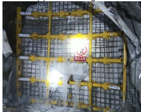
(c) Assembled retaining wall with metal components
