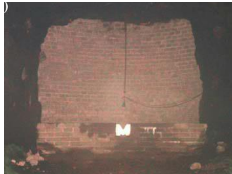
(b) Brick retaining wall
